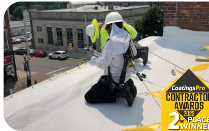
Spray-Tec, Inc. won 2 nd place for the “Ohio Theatre Renovation” project.
