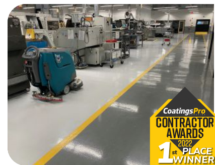
C.A. Reed Associates won 1 st place for the “Horst Engineering Facility Renovation” project.
